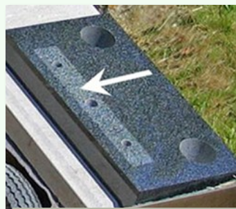
Mating surfaces should be roughened to ensure good adhesion. Water will track under cement placed directly on polished surfaces.
