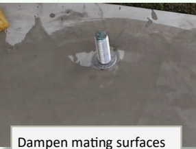
Dampen mating surfaces
