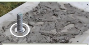
Fully bed the joint leaving space around the anchor. When placing the base work the joint to spread the cement and remove voids.
